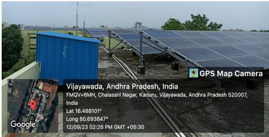
Solar Energy - 200 kW Rooftop Installation and Wheeling to the Grid with APCPDCL
